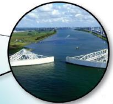
Surge Barrier Gates
